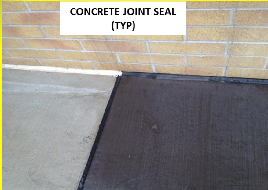
BLDG SIDEWALK & CURB POURED IN PLACE
